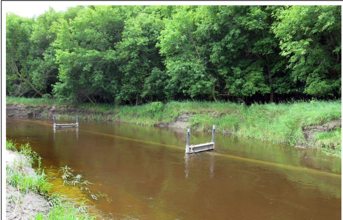
Exposed Enbridge crude oil pipeline in the Tamarac River in Marshall County, MN. (Photo: Dan Gunderson/MPR News)
